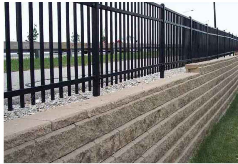
TUBE STEEL FENCE ON CMU BLOCK RETAINING WALL. REFER TO CIVIL ENGINEER'S PLANS FOR WALL HEIGHT.
