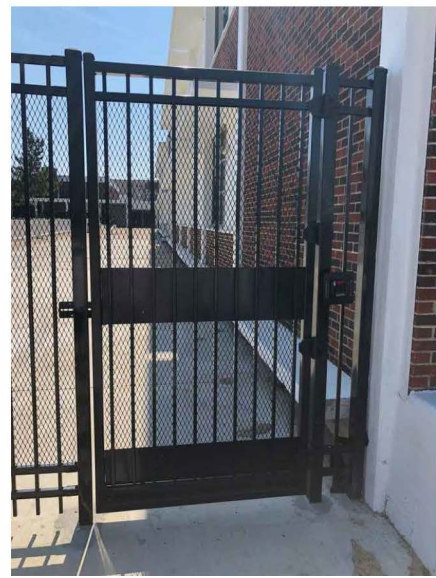
6' TUBE STEEL PEDESTRIAN GATE
