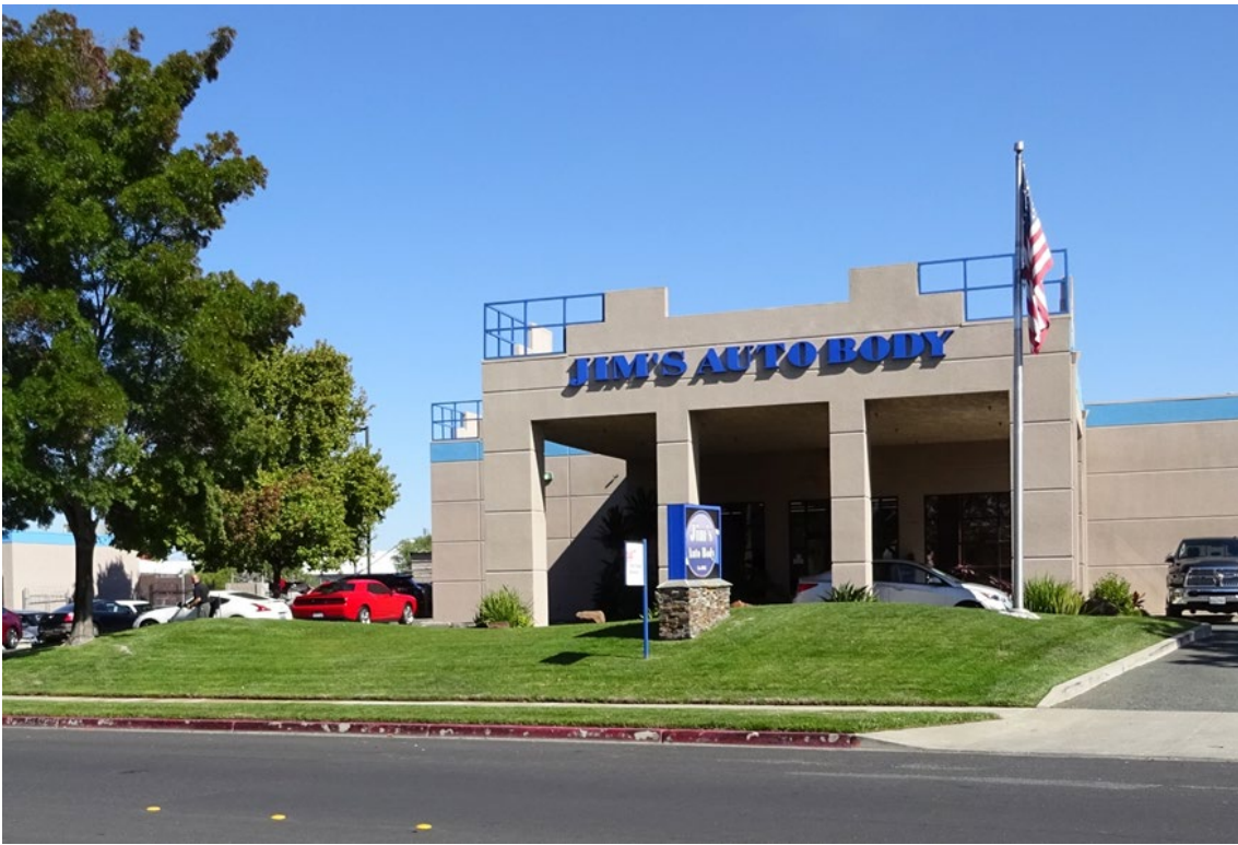
1401 Verne Roberts Circle (existing Jim's Autobody location)
