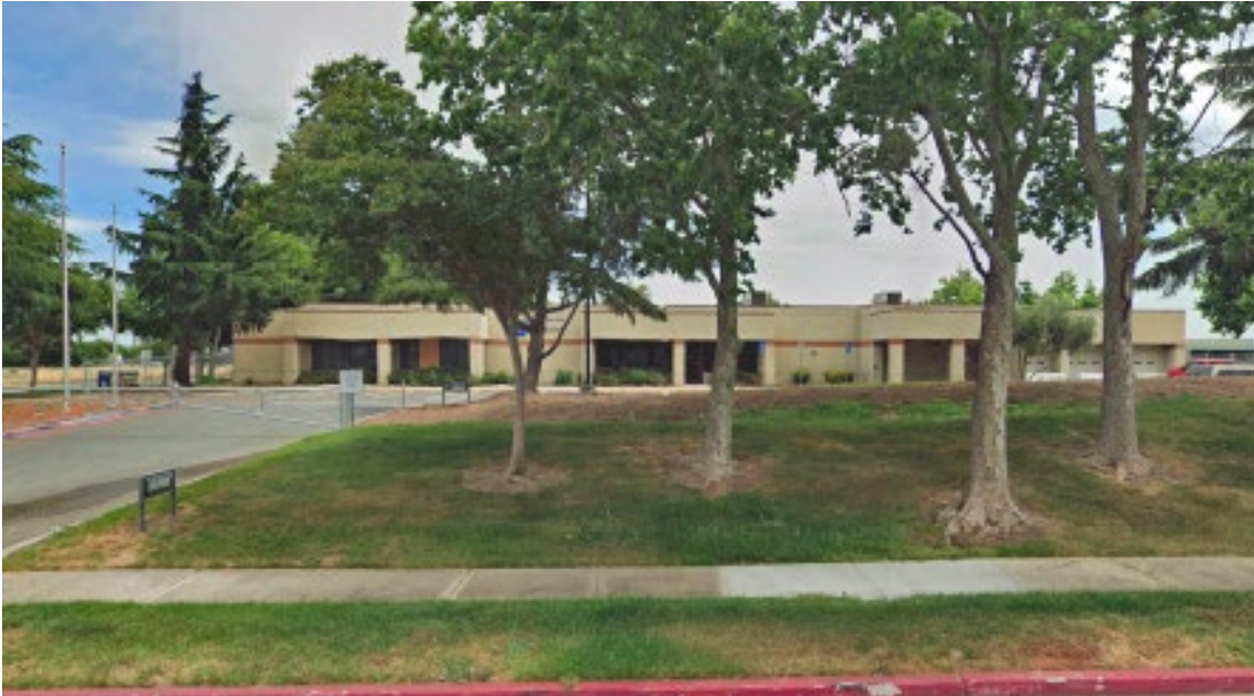
1901 W. 10 th Street (Google Street view 2018)
