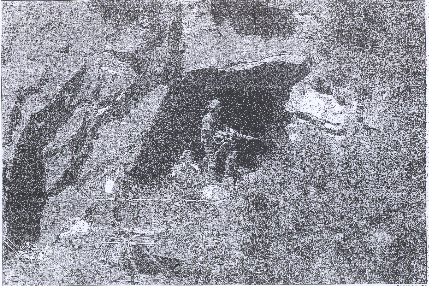
NOZZLEMAN Randy Dutton sprays shotcrete into a mine opening near Coal Canyon while working on the Nortonville Maintenance Project at Black Diamond Mines Regional Preserve.
